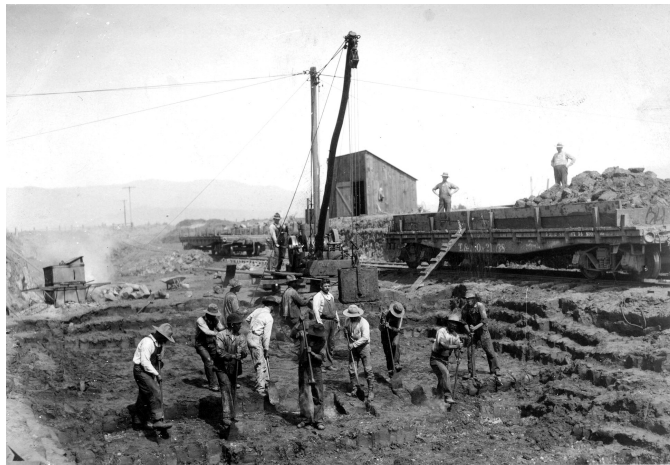
Workers used iron spades heated in a box furnace to cut through rock asphalt at the Las Conchas mine, c.1895. Museum archive photo.
